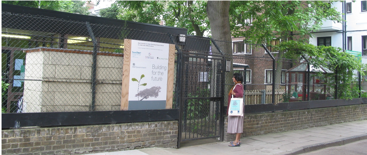
Existing entrance gate, boundary wall and fence
