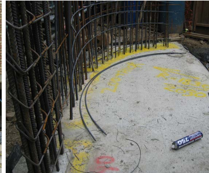
Reinforcement to the curved 'turret' wall
