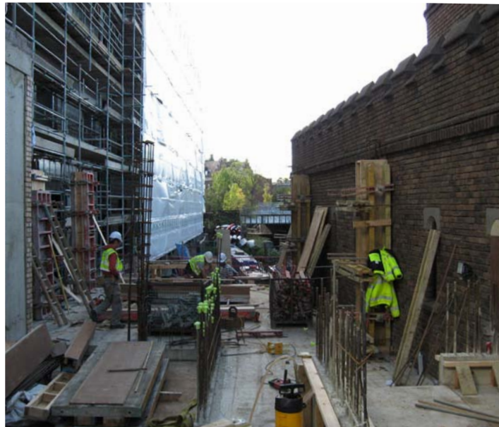
First floor level slab prior to breaking through to the existing
