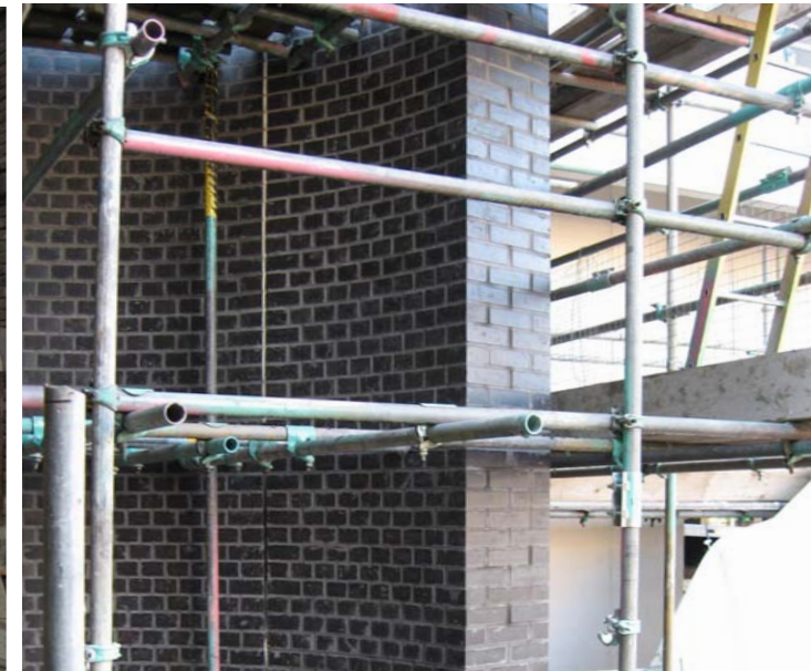
Brickwork cladding to 'turret' wall
