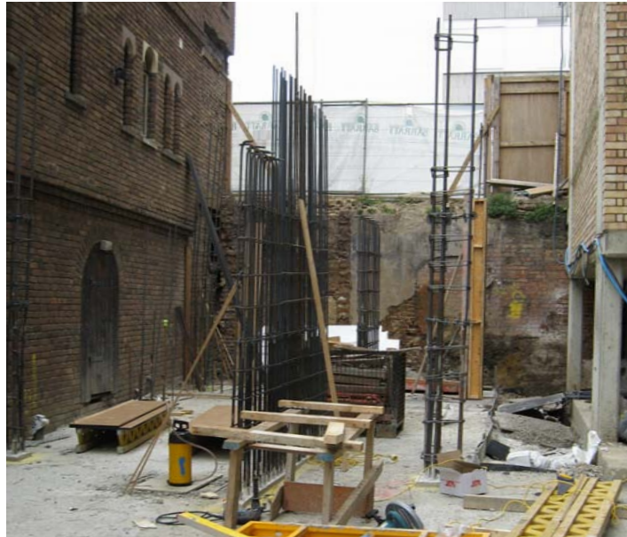
Canal level slab and reinforcement to spine walls
