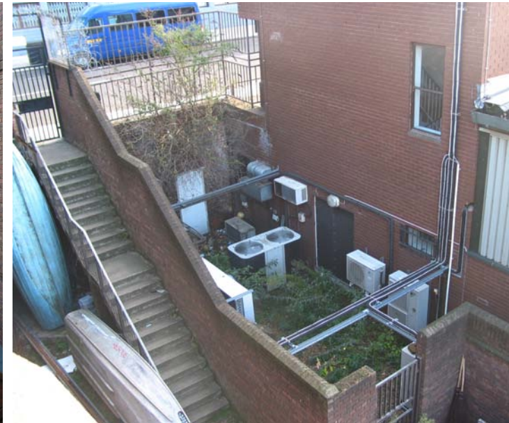
Existing site showing the level change between the street and the canal
